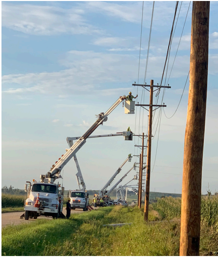
Replacing broken poles in southern Jones County
