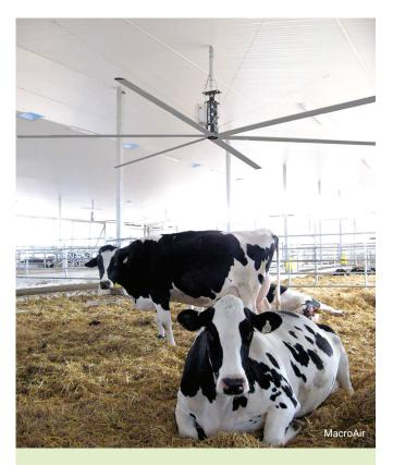
A 24-foot HVLS fan will move as much air as six standard industrial high-speed fans and consume only one-sixth the energy. In a typical dairy-free stall barn, HVLS fans are placed over the feed alley every 35-60 feet, depending on the fan size.
